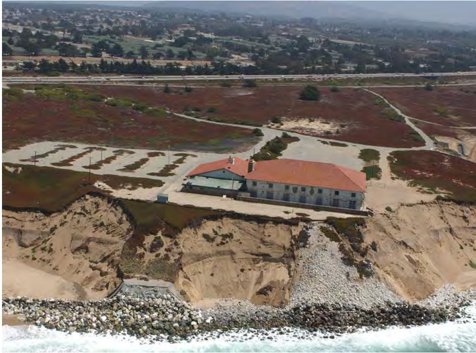
Stilwell Hall, Fort Ord. Facing bluff erosion, this World War II era building was demolished in 2003. Copyright (C) 2003 Kenneth & Gabrielle Adelman, California Coastal Records Project
