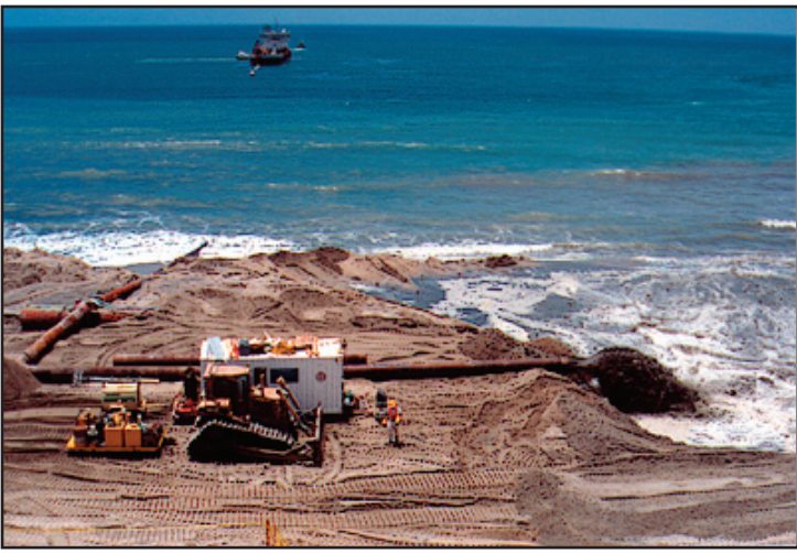
Figure 5.5: Beach nourishment at South Carlsbad State Beach. In July 2001, 150,000 yds 3 of sand were placed on this beach in a fill that was 2000 feet long, 180 feet wide and up to + 12 feet msl.
