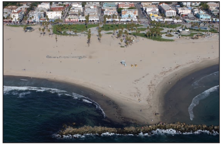
Figure 5.3. Offshore breakwater at Venice where beach has widened in protected area behind breakwater (2004). Photo © Kenneth and Gabrielle Adelman, California Coastal Records Project, www.Californiacoastline.org
