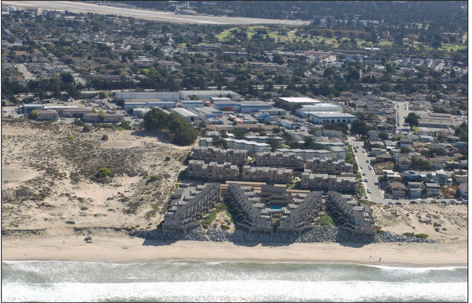
Dune erosion threatens the Ocean Harbor House apartment complex on Del Monte Beach, Monterey CA (October 2005). Copyright © 2005 Kenneth and Gabrielle Adelman, California Coastal Records Project, www.Californiacoastline.org .
