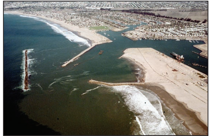
Figure 3.8: Ventura Harbor: maintenance dredging in 1972. Copyright © Kenneth and Gabrielle Adelman, California Coastal Records Project www.Californiacoastline.org
