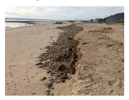
The cobble berm at Surfers' Point, buried beneath the sand, extends beneath the dunes back to the bike path. The berm, which is up to eight feet thick, provides a significant mass of natural river rock to protect the bike path from extreme events and future sea level rise.
