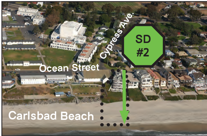
SD # 2 - Beach Access Stairway, 2601 Ocean Street, City of Carlsbad. OTD recorded 1983. Permit # A-77-81 for three condominium units.
