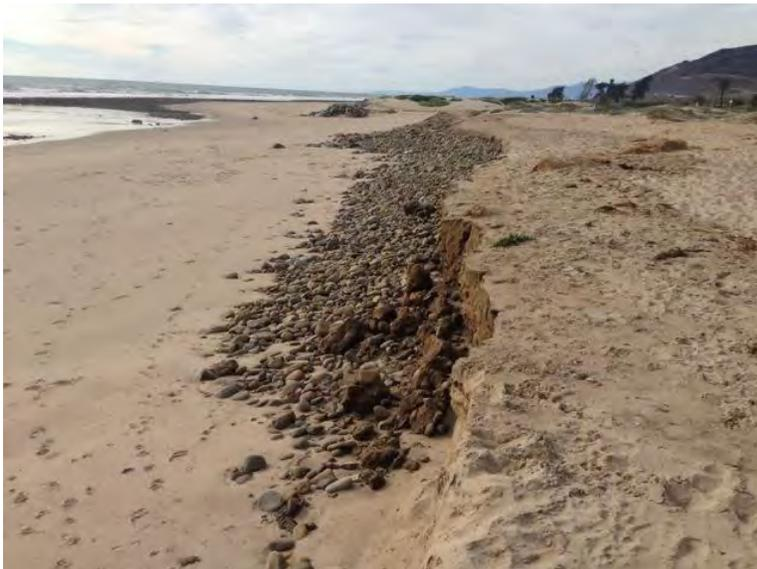
*The cobble berm at Surfers' Point, buried beneath the sand, extends beneath the dunes back to the bike path. The berm, which is up to eight feet thick, provides a significant mass of natural river rock to protect the bike path from extreme events and future sea level rise.*
